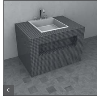
C Tiling of the bathroom furniture can be carried out.
